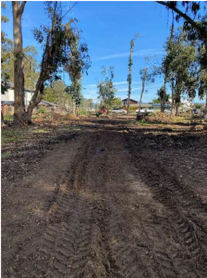
During Tree Removal – June 2025
