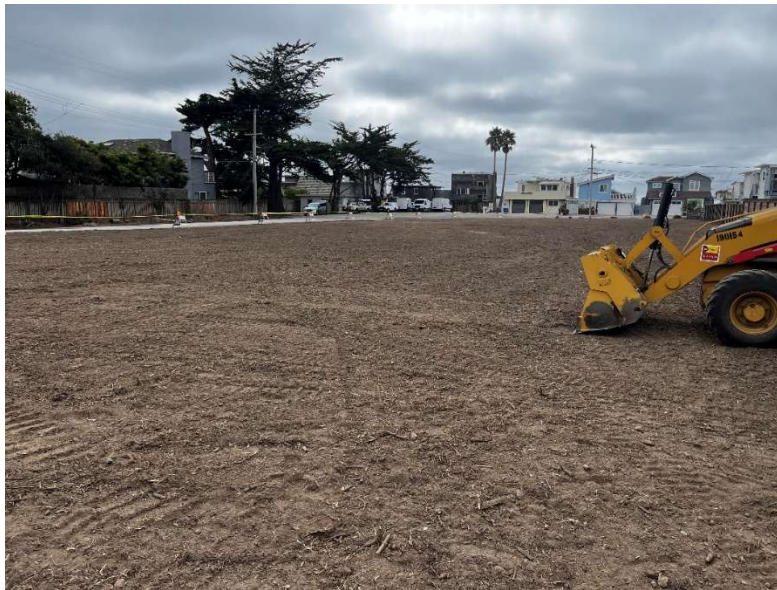
Grading Complete – October 2025
