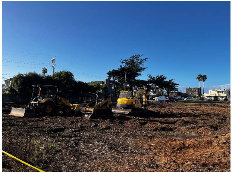
During Grading – September 2025
